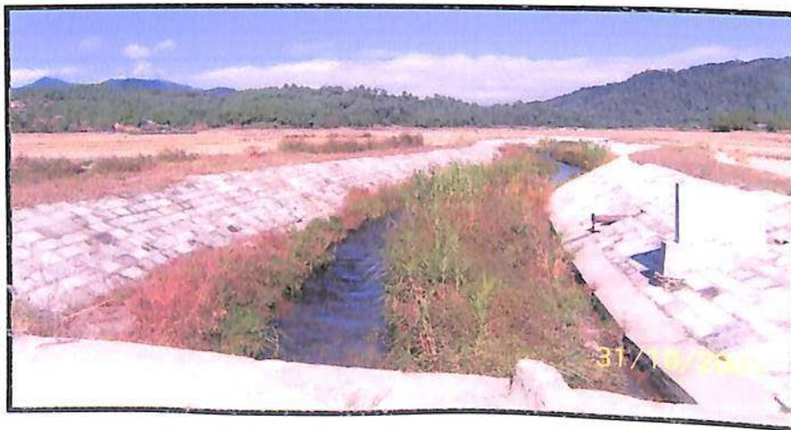
Plate No.18: Soil erosion control measures adopted along the Kiile River
