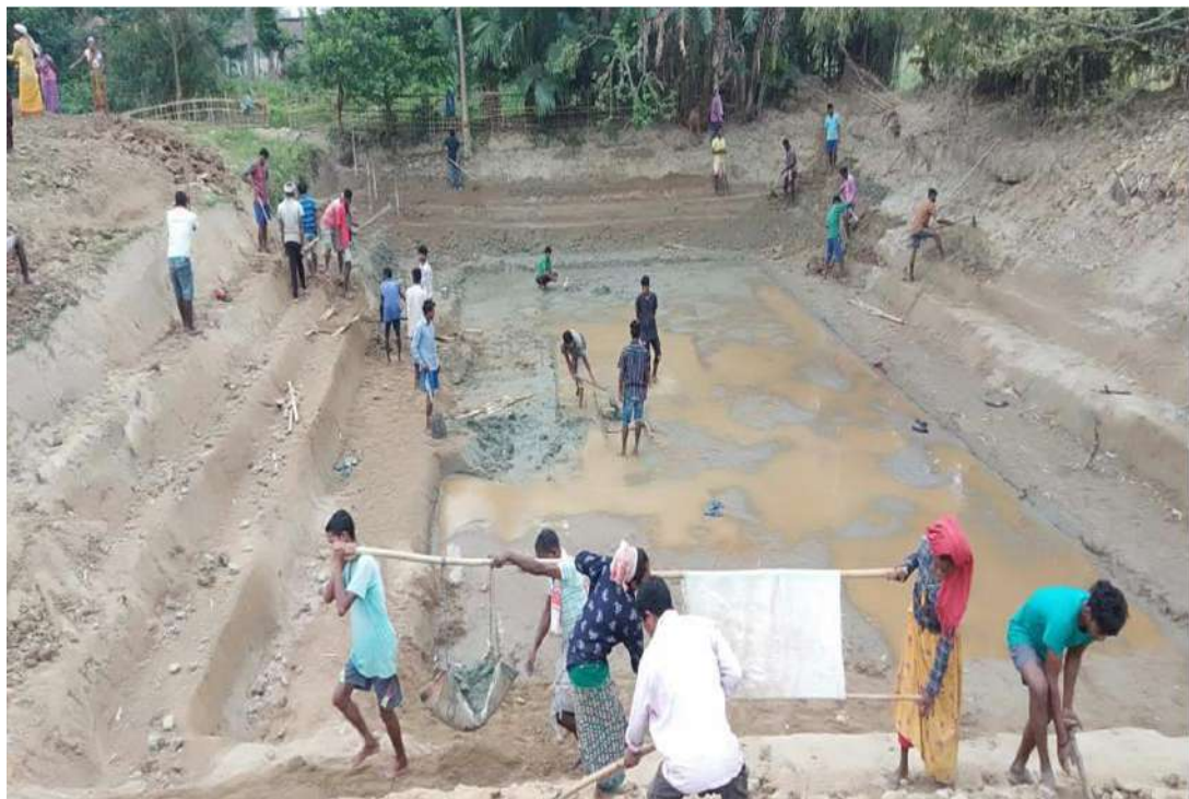
Construction of Farm Pond at Lekang CD Block, Namsai District
