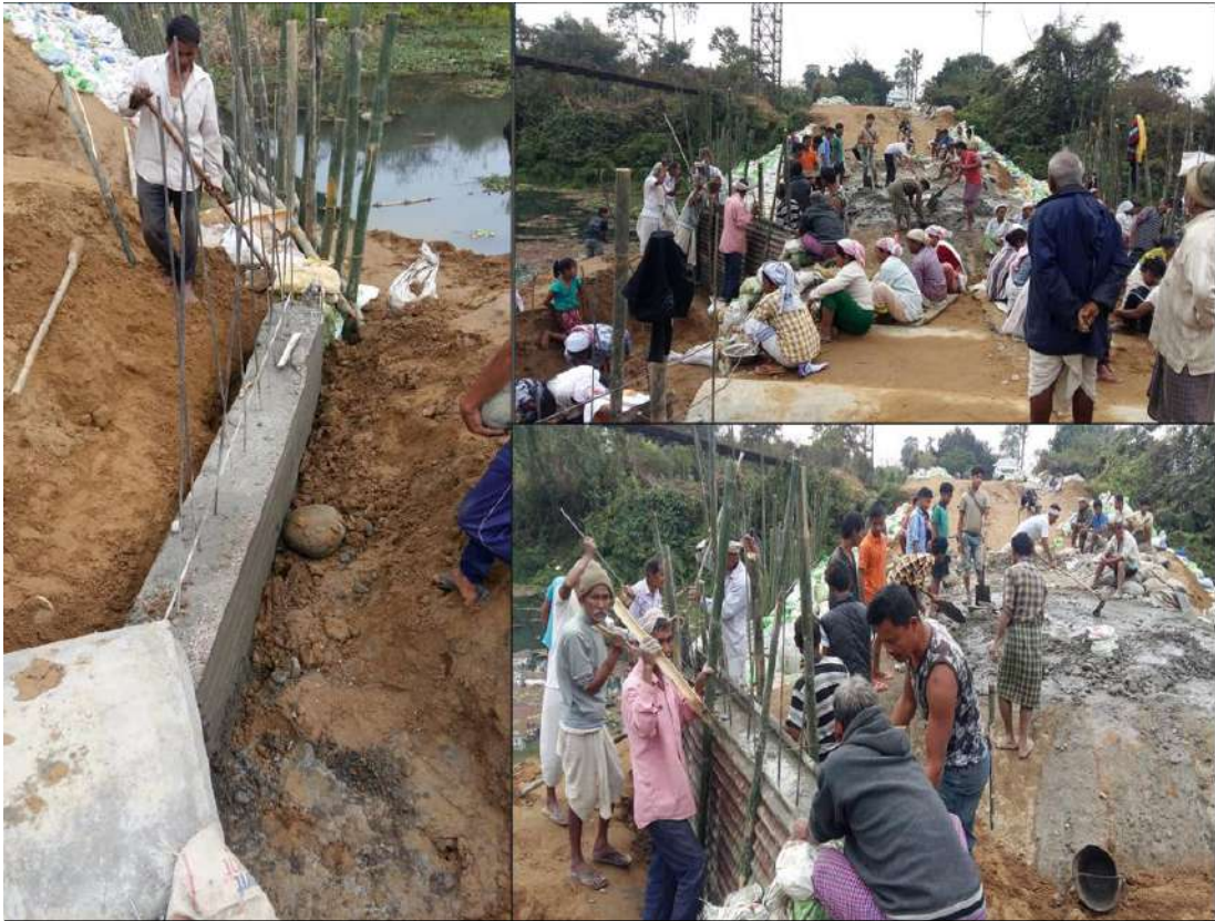
Construction of Flood Protection at Lekang CD Block, Namsai District
