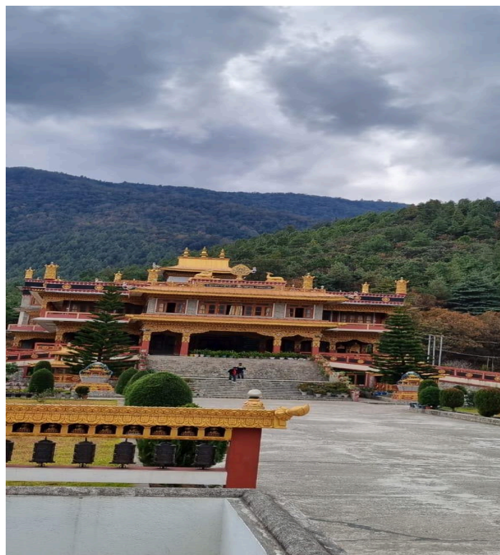
Pic 3.50: Outside view of Thupsung Dhargye Ling Monastery at Dirang.
