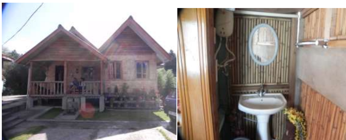
Fig. 7. Homestay facility in Ziro valley
